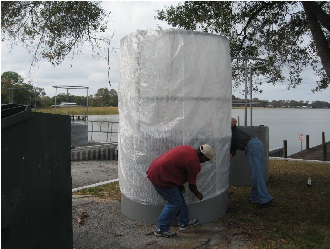
a. Reinforced Bag is Placed Over the Aluminum Cylinder and Ring
