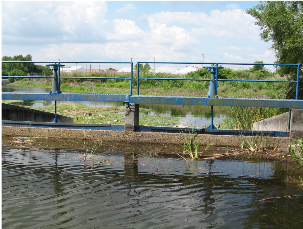
a. Primary Weir Structure
