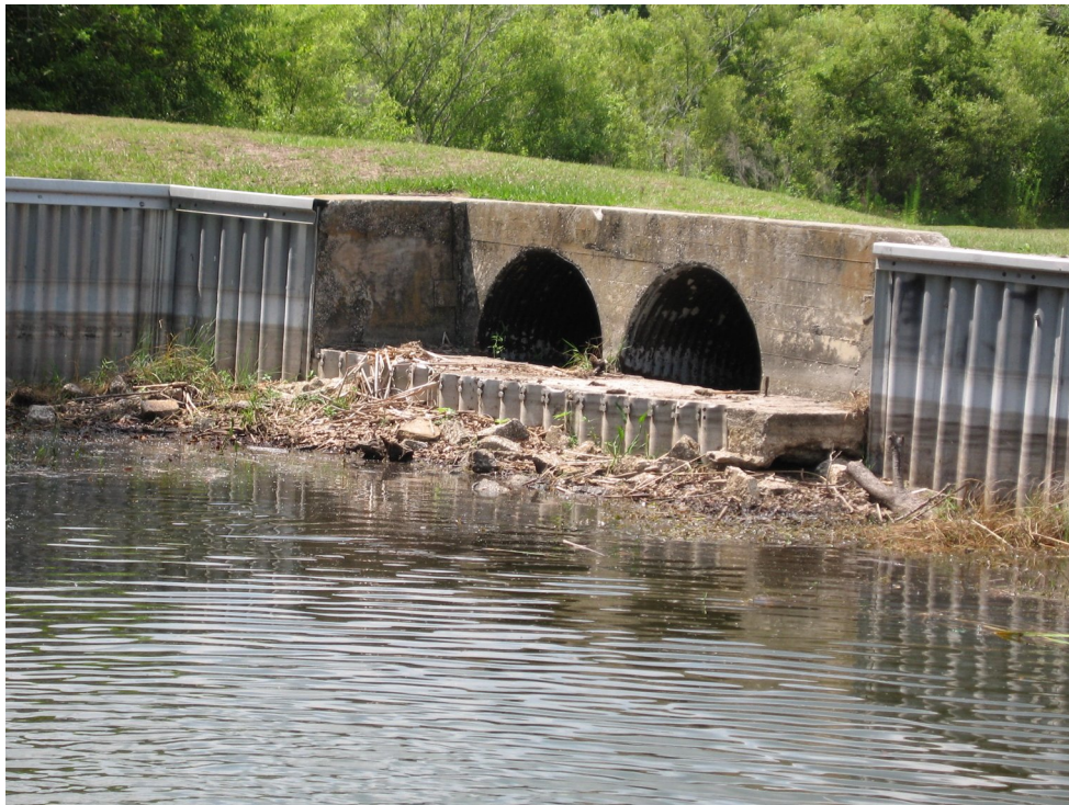
b. Supplemental 24-inch RCP Outfalls
