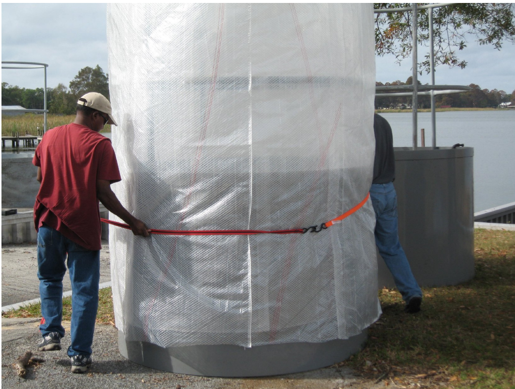
b. Bag is Secured to Bottom Cylinder Using a Ratchet Strap
